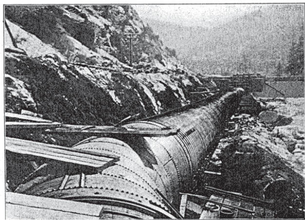
FIG. 2.—RIVETED STEEL ELBOW IN 9-FT. REDWOOD PIPE, NEAR FLORISTON, CAL.
