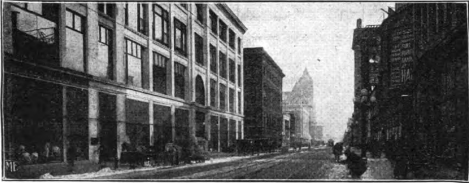
WOOD BLOCK PAVING ON HEAVY TRAFFIC BUSINESS STREET.
