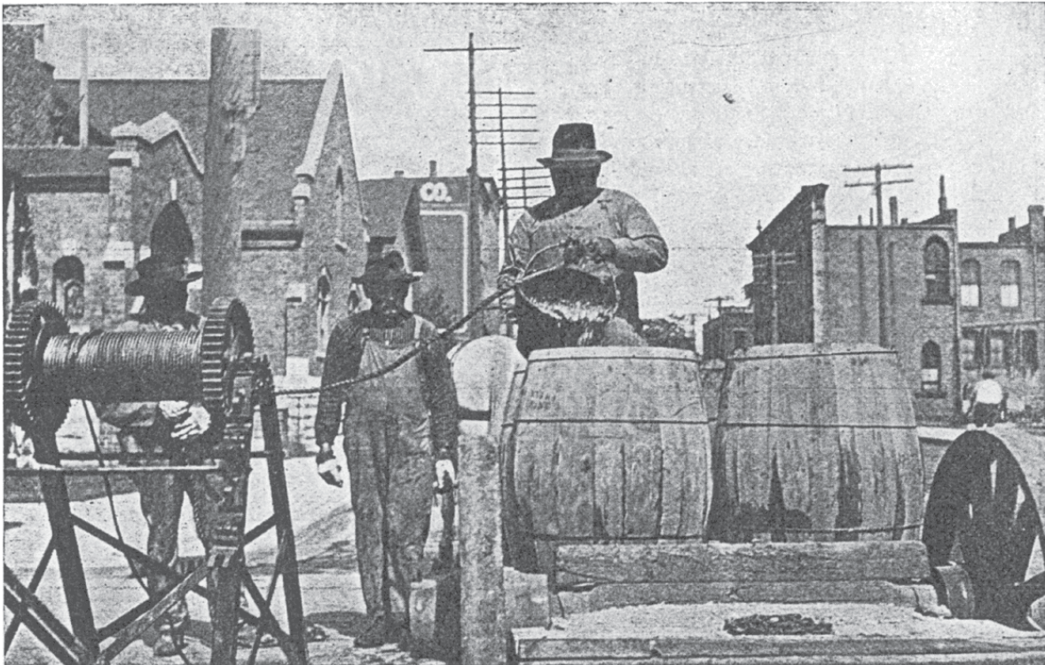
TURBINE SEWER CLEANING machine removing tar from a sewer at Fond du Lac, Wis.
