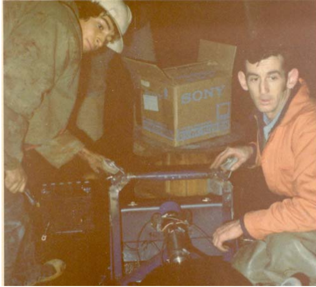
Figure 6. Lowering early inspection camera Source: Pipe Recon Services, Surrey, BC.
